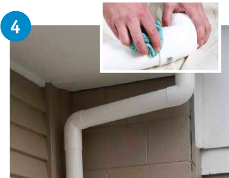
4 Solvent cement all remaining elbows to downpipe on ground, before completing offset installation.
