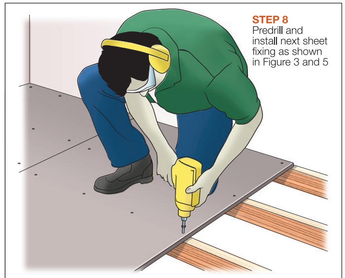
FIGURE 11 PRE DRILL NEXT SHEET
