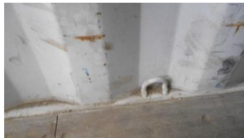
Example of tie-downs used throughout container
